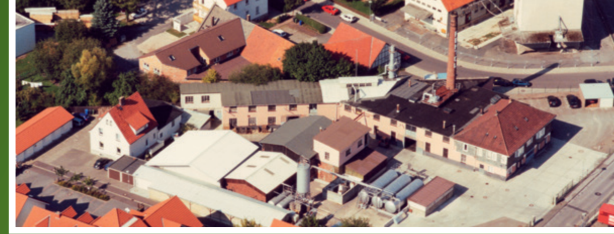
Luftbild 1988 Aerial photograph 1988
