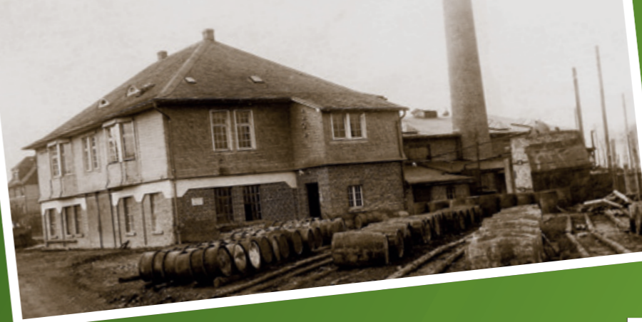
Fabrik-Neubau in Korbach 1907 New factory building in Korbach 1907
